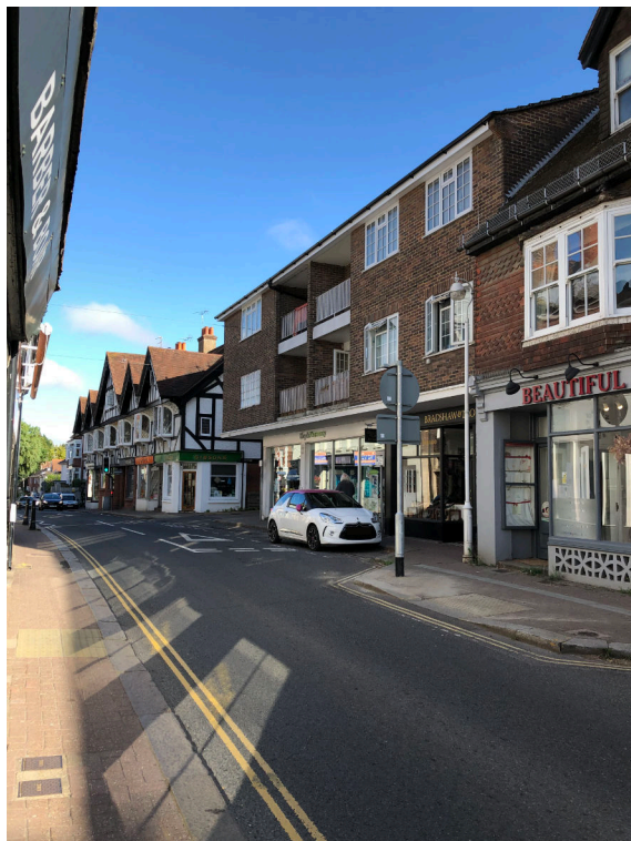
Village High St. block of flats, shops and parking
