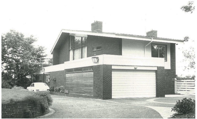
The Long House, Langton Lane
